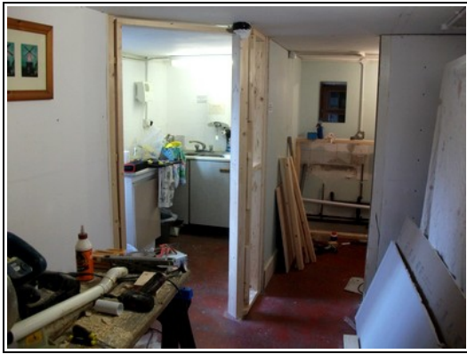
Work in progress (above)
